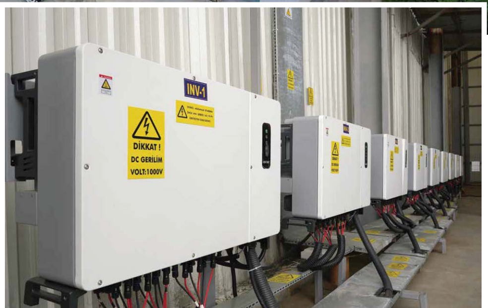
9 units of PVISU3-125KI powering a mineral water factory (1MW)
